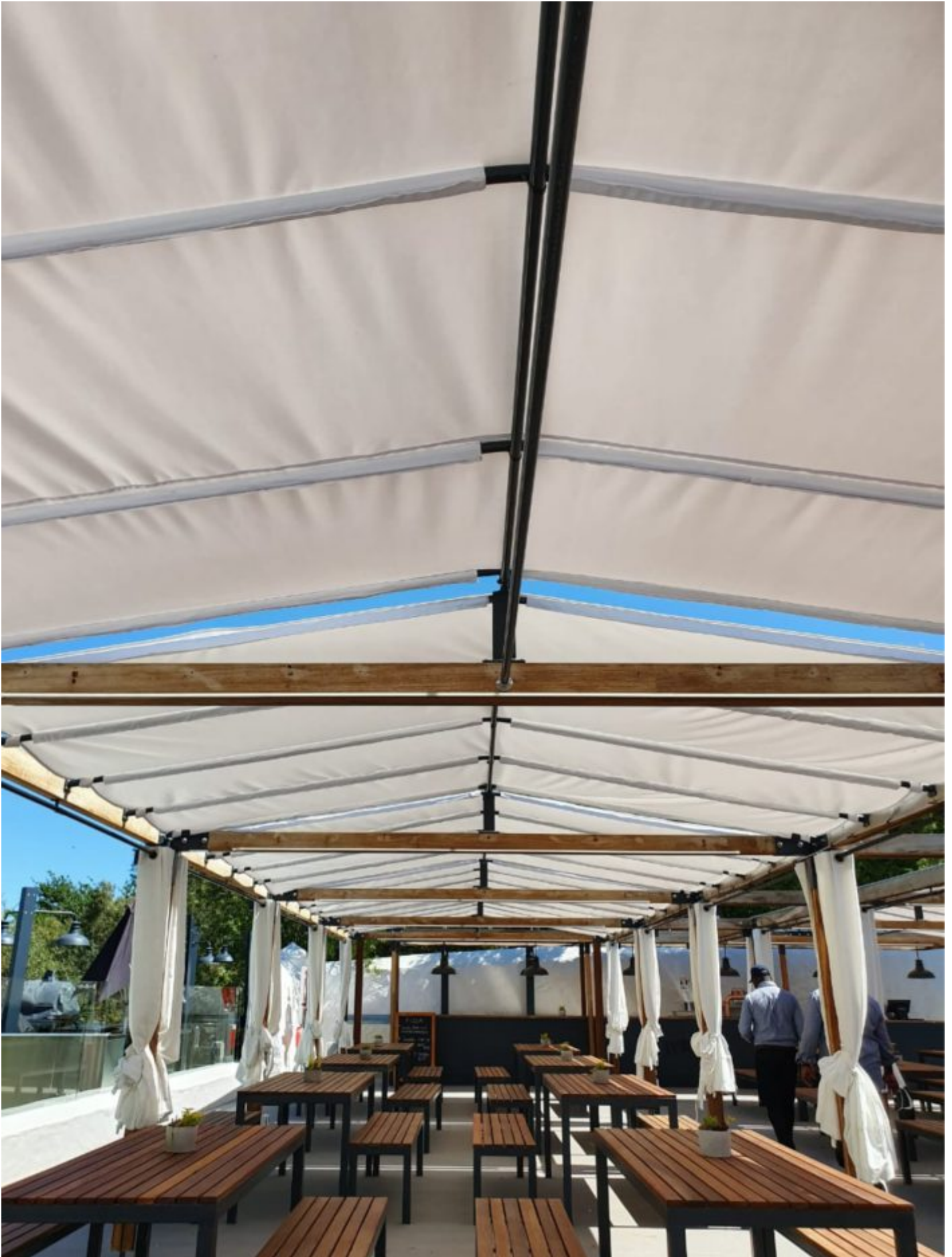
THE KRAAL: Purpose Built Gazebos using Kiaat posts and beams with Steel Support connectors, finished with waterproof canopies attached to an aluminium structure and Shear weave curtains. Custom size benches and tables with steel frames and slatted hardwood tops.
