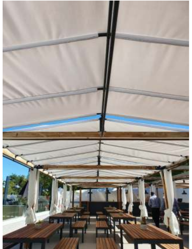
BRIEF: Manufacture and install 10 purpose built Gazebos using solid Kiaat posts and beams with Steel Support connectors, complete with waterproof canopies attached to a aluminium roof trusses and finished with shear weave curtains. Furnish with custom made steel tables and benches, finished with recycled kari wood slats, sealed with Timbercare.
